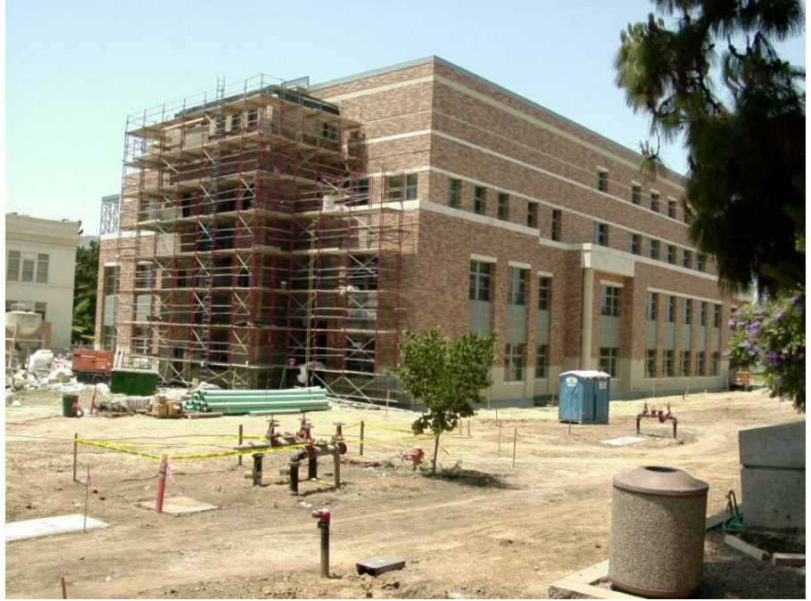
Chapman University: Almost finished
