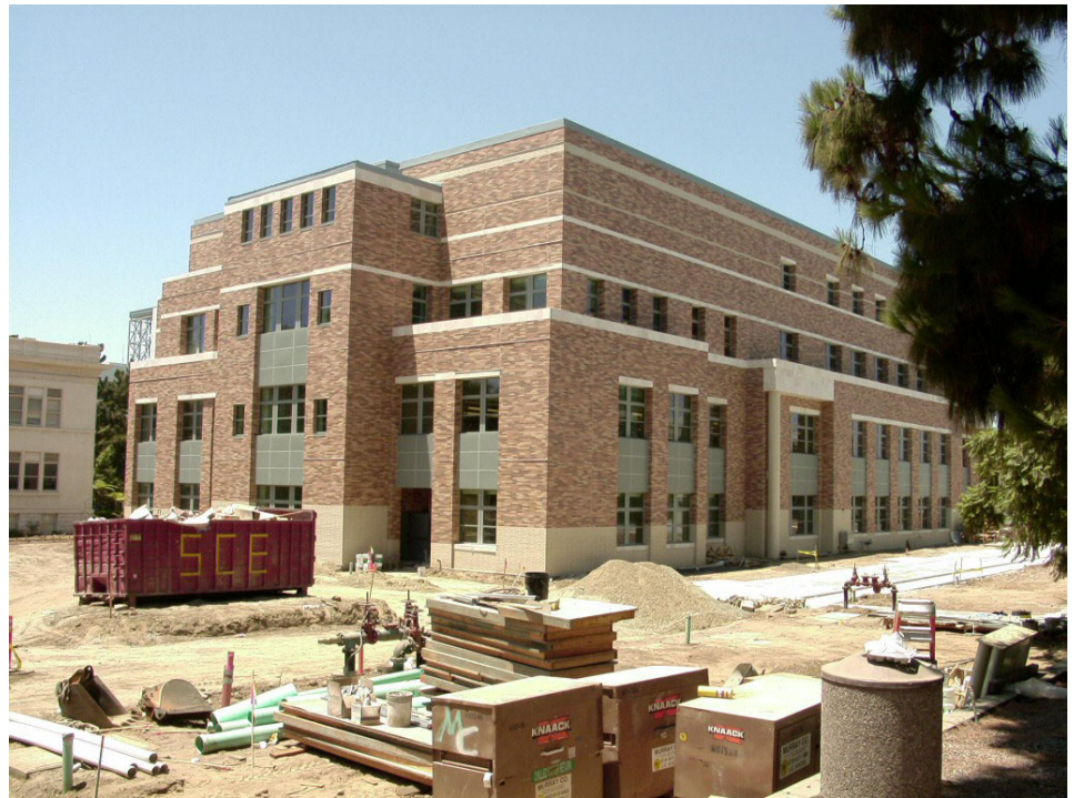
We can see lights in the new building now
