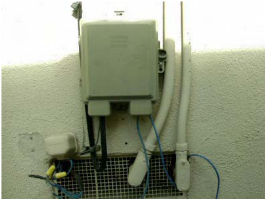
The outside box and the master splitter installed
